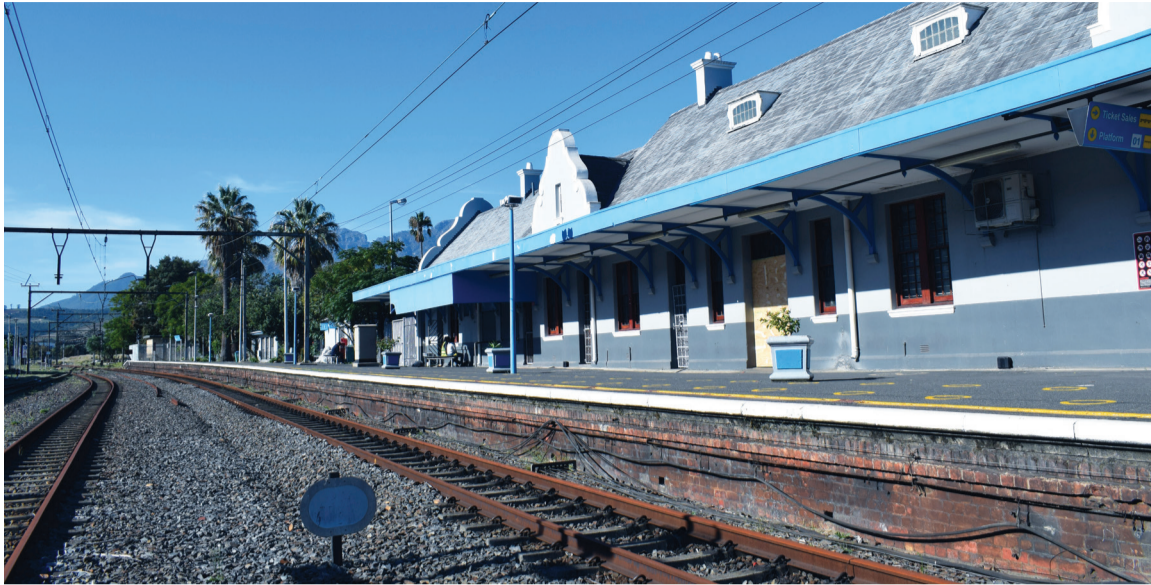
The Stellenbosch train station is on the Northern Line train route that is currently not fully operational. This poses problems for commuters in the Cape Winelands area, according to Zinobulali Mihi, the acting marketing and communication manager of Passenger Rail Agency of South Africa. Photo: Kirsty Bucholz
